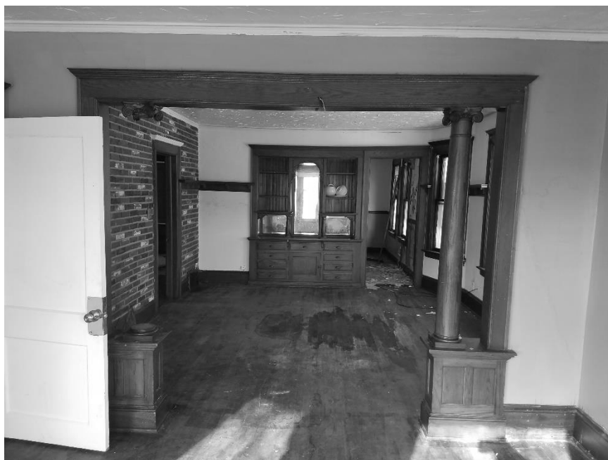
Figure 2. Interior of vacant duplex in Milwaukee.
