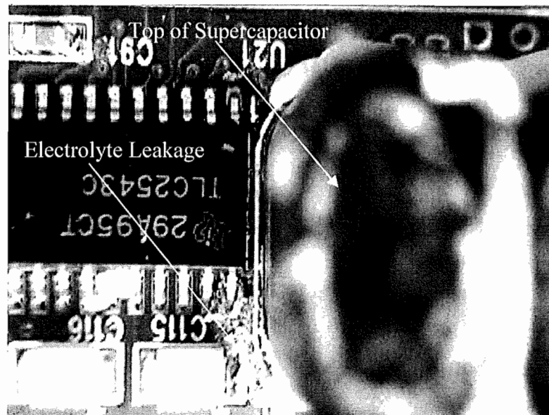
Figure 4. Photo showing supercapacitors electrolyte leakage on company XYZ's product
