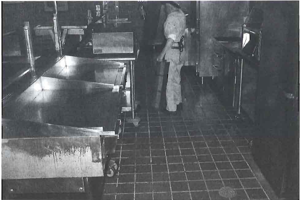
Photo of the fryers with a greasy film on the floor surface.
