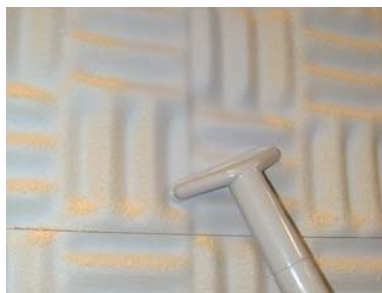
Figure 4.5. Photograph of cleaning SONEX foam with standard vacuum and attachment demonstrates level of cleanliness.
