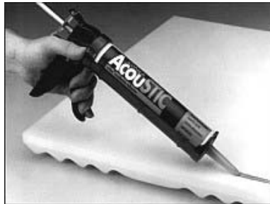
Figure 2.1. Application of acoustical foam using SPA-02 adhesive (Illbruck, 1998).
